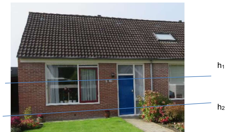
Figuur 7: Bepaling van percentage openingen in langsgevel.
